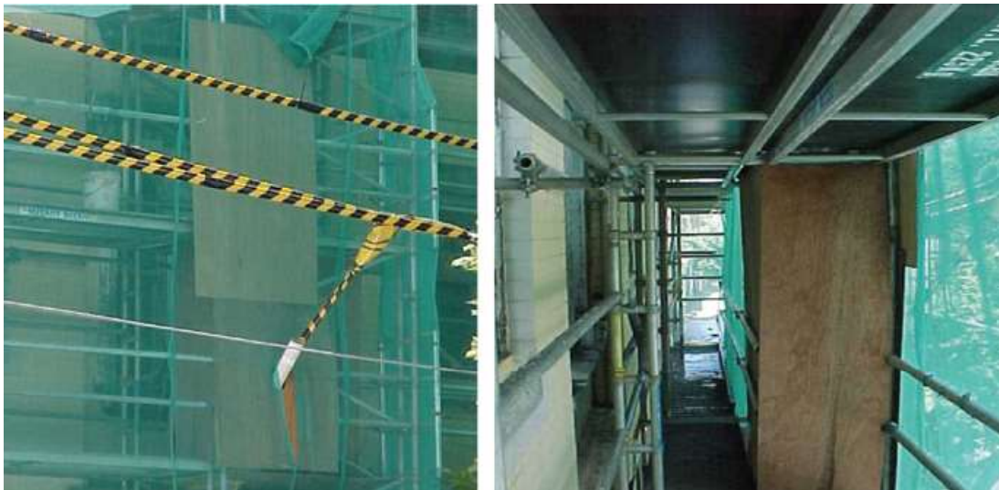
Figure 11 – Enclosure of overhead powerlines
