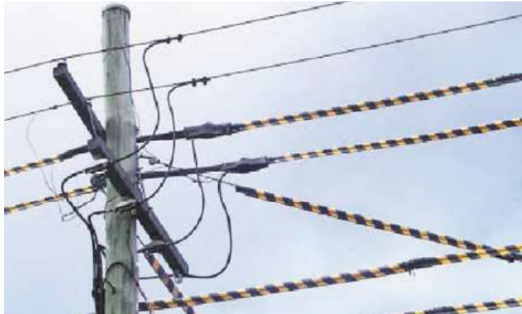
Figure 16 – Tiger tails fitted to overhead power lines
