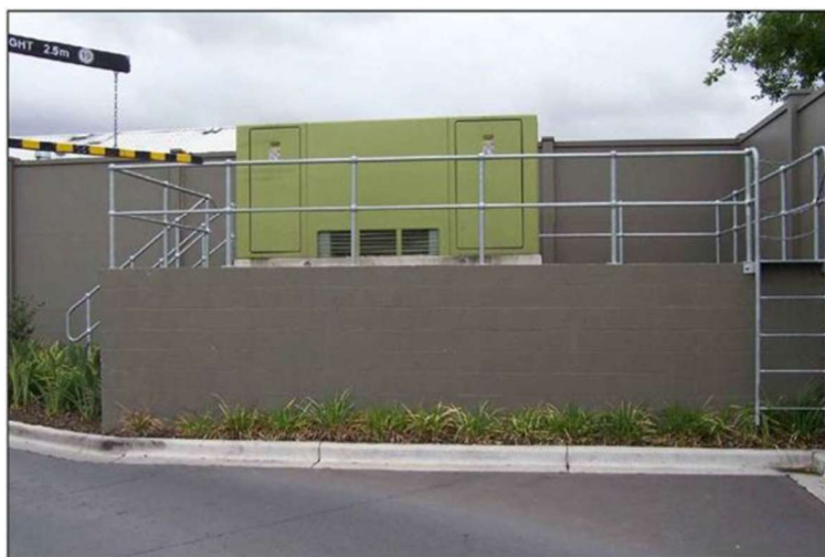
Figure 51 - Example substation raised above 1:100 flood level
